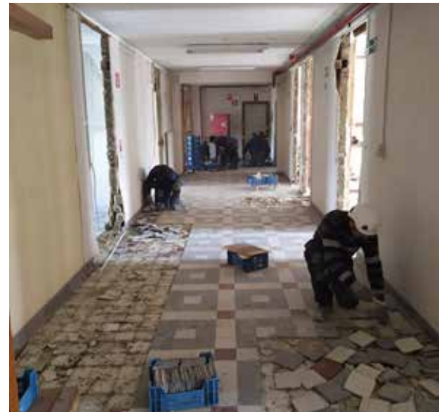
Recovery of hydraulic tiles in a demolition. Source: Rotordc www.rotordc.com
